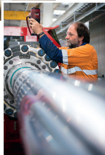
From the dismantling area to the reassembly area, compressed air is used to power large torque and rattle guns, grit blasting as well as the painting booth.
